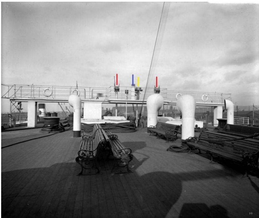
Olympic after docking bridge. (Red, docking telegraphs; blue, steering pedestal [w/o wheel]; yellow, compass). Credit: Wiki Commons
